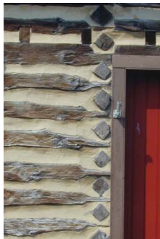
Exposed logs show the construction of the building..
