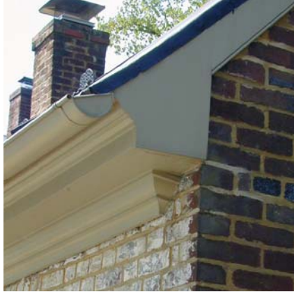
A simple wood cornice and boxed eave.
