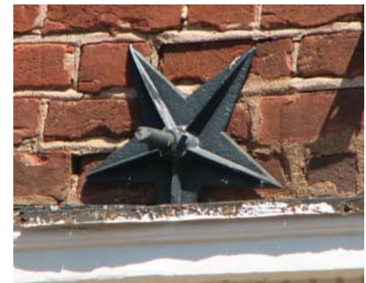
Metal structural ties are a functional feature that may also be decorative.
