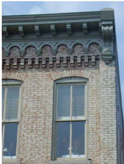
An wood Italianate bracketed cornice decorates this commercial building.
