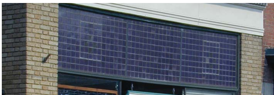
An original prismatic glass transom window located above the storefront windows diffuses the light and helps to illuminate the store interior.
