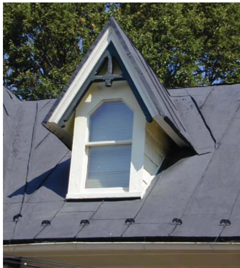
Metals are most commonly found in roofing and gutters.
