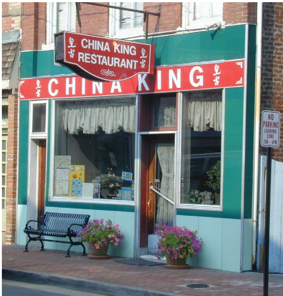
A recently rehabilitated example of a pigmented glass storefront. These glass panels in different colors were a very popular cladding for storefronts in the mid-twentieth century.
