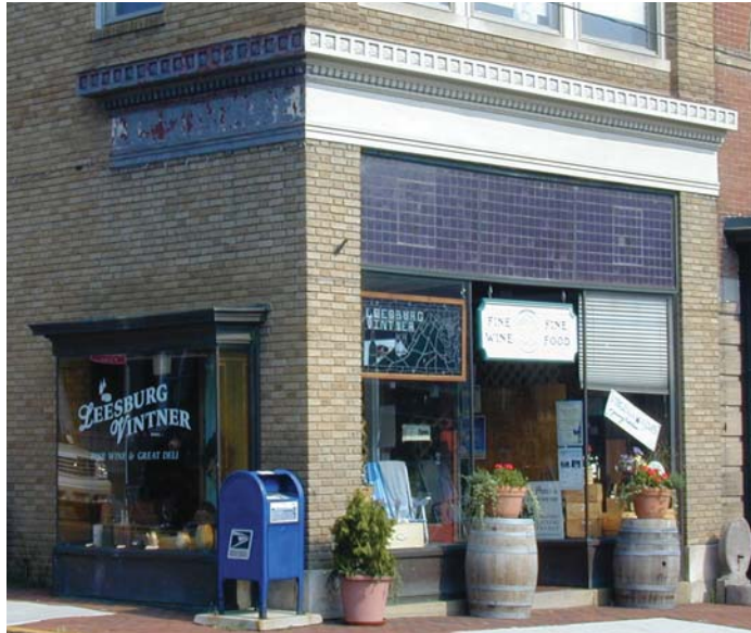
This metal cornice, storefront, and box bay display window illustrate the use of metal as a practical and decorative material.
