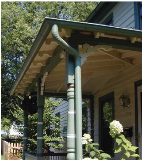
A wood porch with turned columns, decorative brackets and exposed rafter tails.
