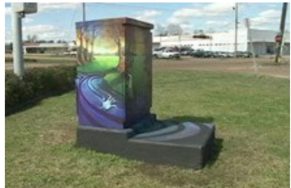
Artwork on utility boxes
