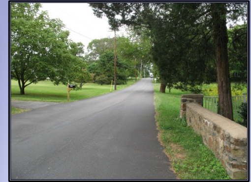
Looking north – north of William Street
