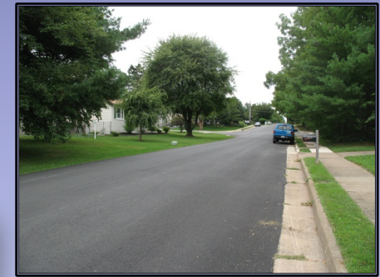
Looking south toward Ayrlee Avenue
