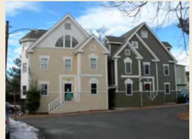
New construction on Wirt Street.
