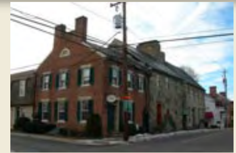
Early 19th century brick building with new construction (the stone buildings) adjacent.
