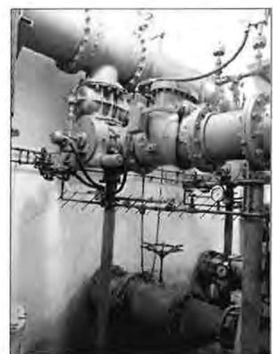
IMAGE - SEAL WATER PIPE NTS
