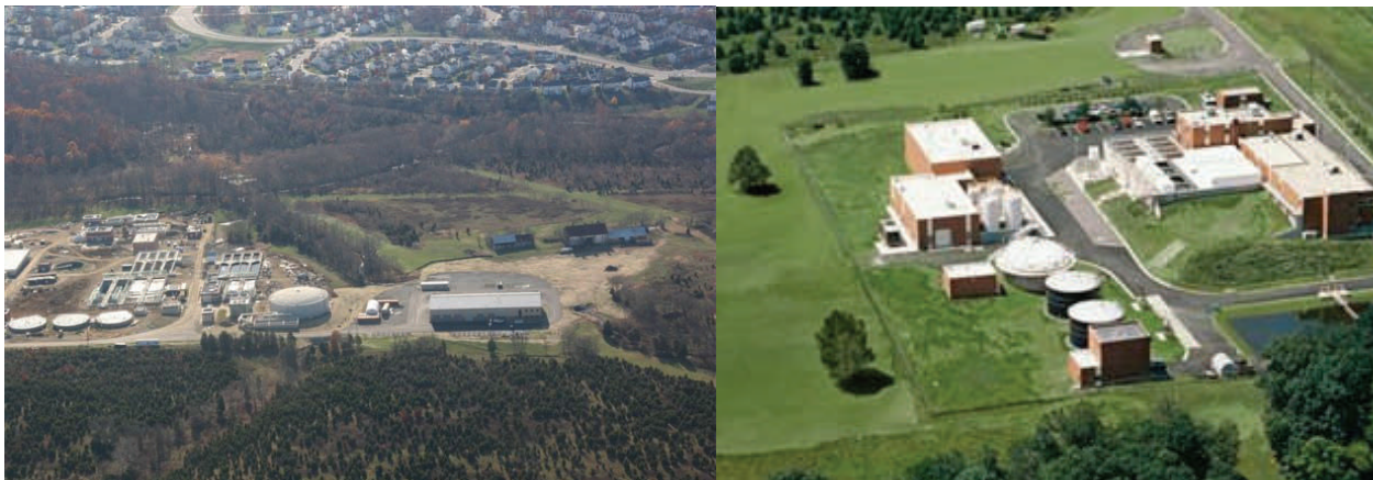
Water Pollution Control Facility and Utility Maintenance Building
