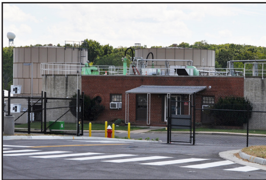
Water Pollution Control Facility Entrance
