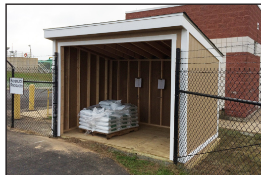
TLC Shed on Russell Branch Parkway
