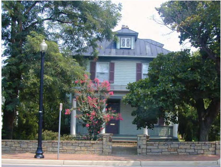
This typical American Foursquare example displays an asymmetrical arrangement of openings, full-width porch and hipped roof. A hipped roof dormer is accented by a pair of diamond-paned casement windows.
