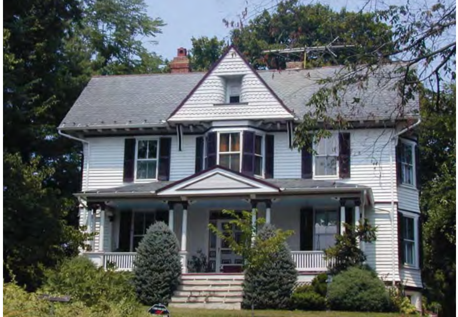
Accentuated by projecting gables over the front door and on the side of the house, this I-house has decorative details which link it to the Queen Anne style. Its symmetrical composition and classical porch columns also link it to the Colonial Revival style.
