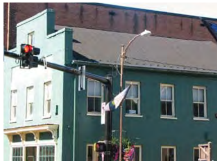
The majority of Leesburg's traditional commercial buildings have gable or hipped roofs; some are hidden behind parapet walls.
