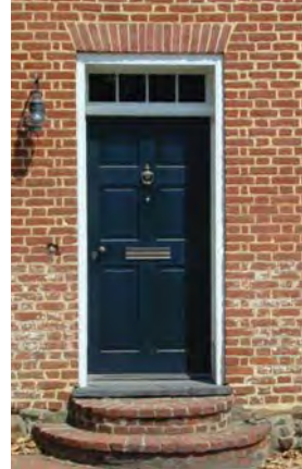
A six-paneled door with a transom above is typical of the Georgian and Federal styles.
