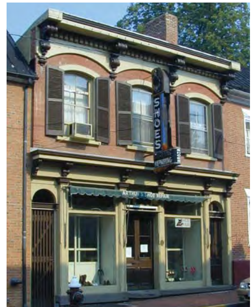
Appropriate shutters fit the opening, as these arched shutters fit the arched windows.
