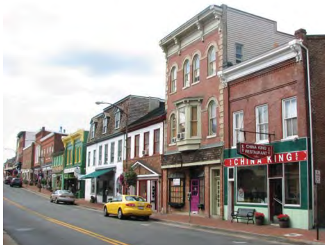
These King Street facades display a variety of roof forms including Mansard, gable and shed.
