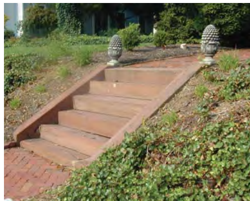
Historic walkways are often constructed of brick. Stairs which lead from the walkway to the sidewalk may be an important character-defining site feature and should be retained.
