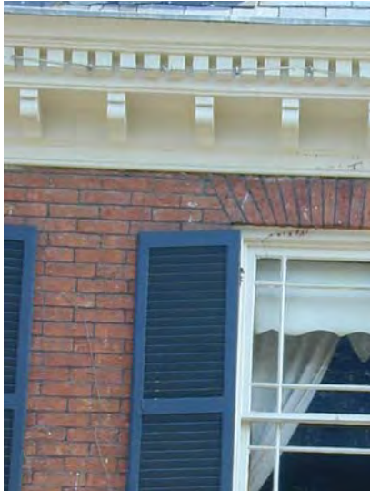
Two very different cornices on residential buildings: a classical dentilated cornice with modillions (left) and a simple, brick, corbeled cornice (above). Both are appropriate to the building's style.
