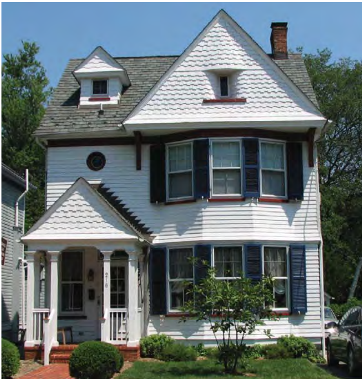
A well-coordinated paint scheme can highlight decorative woodwork such as the gable end fishscale shingles and porch post brackets seen in this example.
