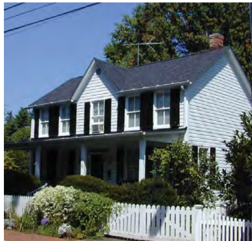
A gable roof with a central gable; the porch has a shed roof.
