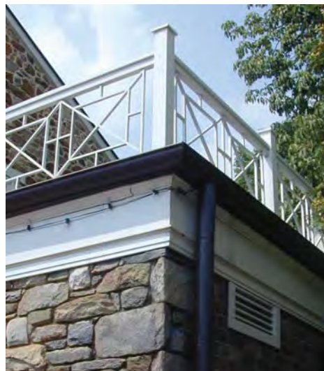
A round gutter and downspout are appropriately scaled to the building, cornice, and other decorative elements.
