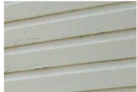
The new German siding (below) replicates the visual appearance of the original material (above).
