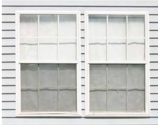
INAPPROPRIATE: False muntins that are flat and clip inside of the glass are not appropriate in the district.
