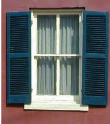
Two-over-two double-hung windows in masonry (above left and middle) and in wood siding with a decorative cap (above right).
