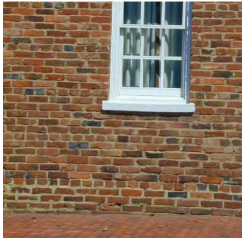
At times the foundation material is the same as the wall material; in this case, a change in brick coursing defines the foundation from the wall.
