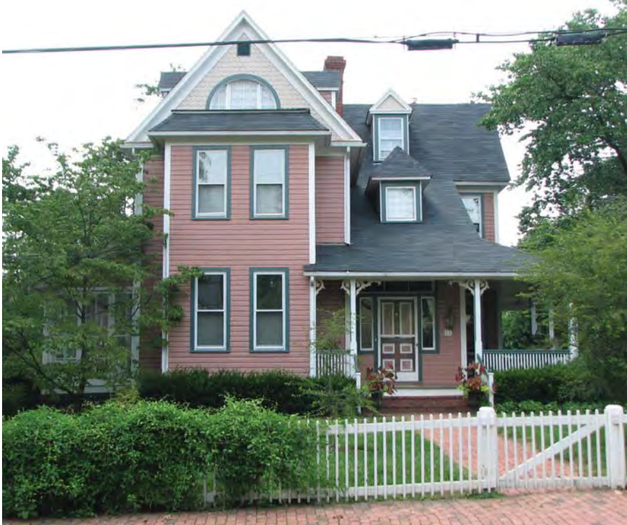
A well-coordinated paint scheme can highlight decorative woodwork such as the gable end fishscale shingles and porch post brackets seen in this example.
