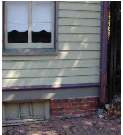
A brick foundation with an original opening.
