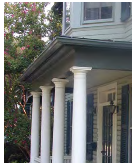
A smaller profile ogee gutter on a residential porch is shown here.
