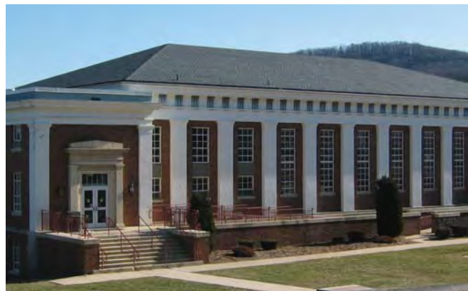
On larger freestanding buildings on bigger sites, which may be more typical for institutional buildings, the design of an accessible ramp can be hidden behind a wall as seen in this example above. A railing that blends in with the building color completes the design.
