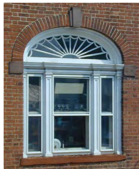
A composite window of one-over-one double-hung windows with a fanlight.
