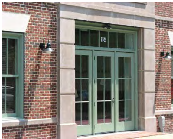
Appropriate commercial building lighting includes historically sympathetic designs such as lanterns and gooseneck fixtures.
