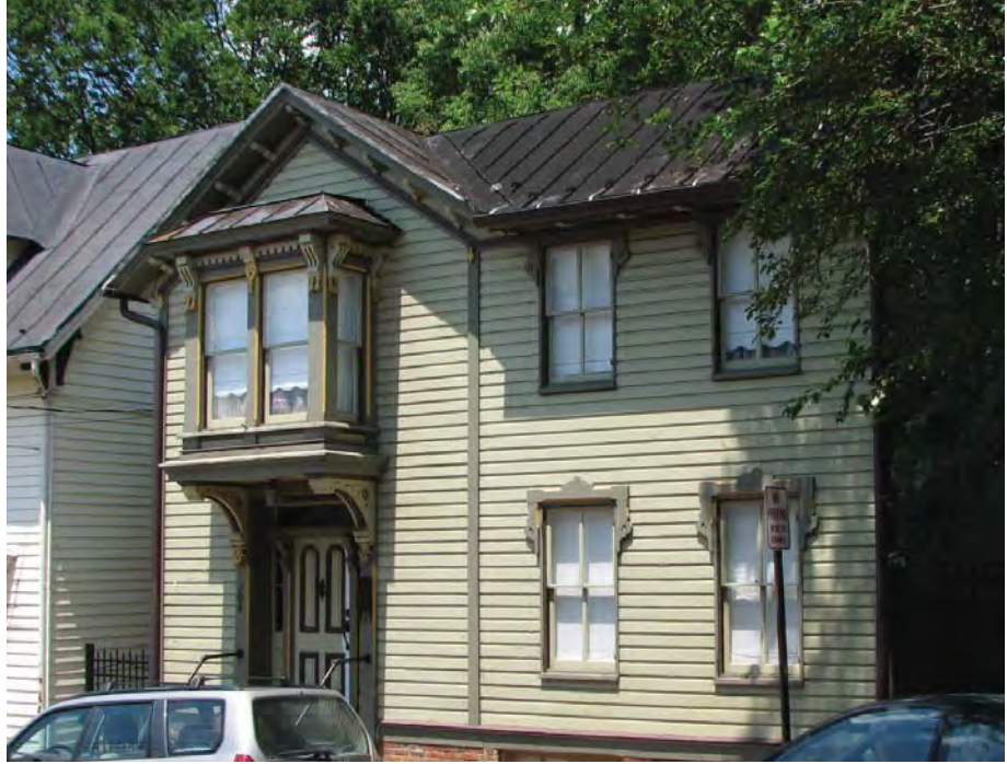
This frame residence displays the projecting bay, bracketed cornice, arched doors, and decorative window molding that are common to Italianate domestic architecture.
