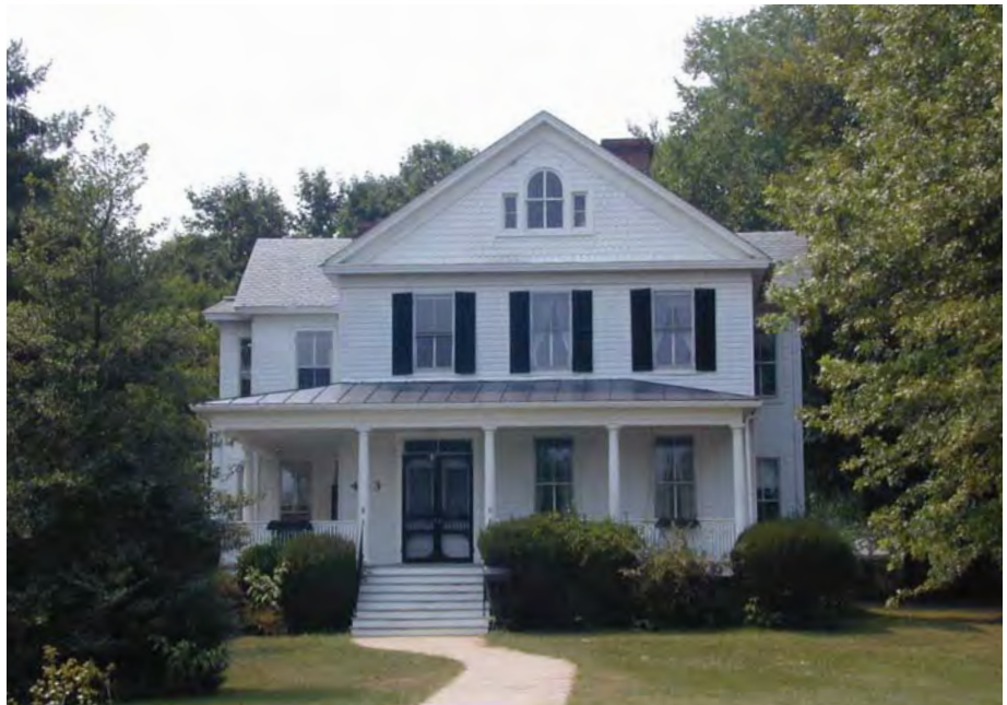
This vernacular example presents its shingled end-gable with Palladian window to the street. A cross-gable projects to the rear of the structure.
