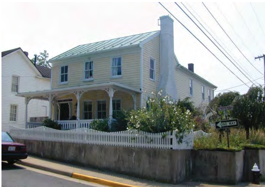
This three-bay vernacular Victorian dwelling with a side-gabled roof, wooden siding, and a full-width porch accented with decorative brackets and balusters is characteristic of the Vinegar Hill neighborhood.
