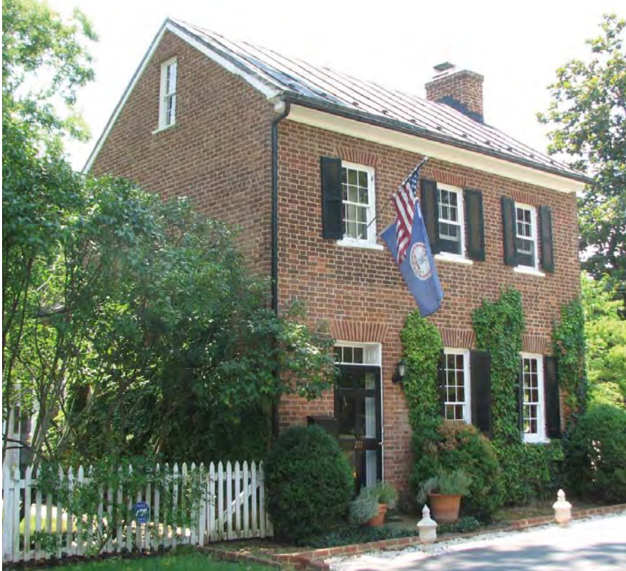
This three-bay Federal-style dwelling features Flemish bond brickwork and jack arches over the window and door openings.
