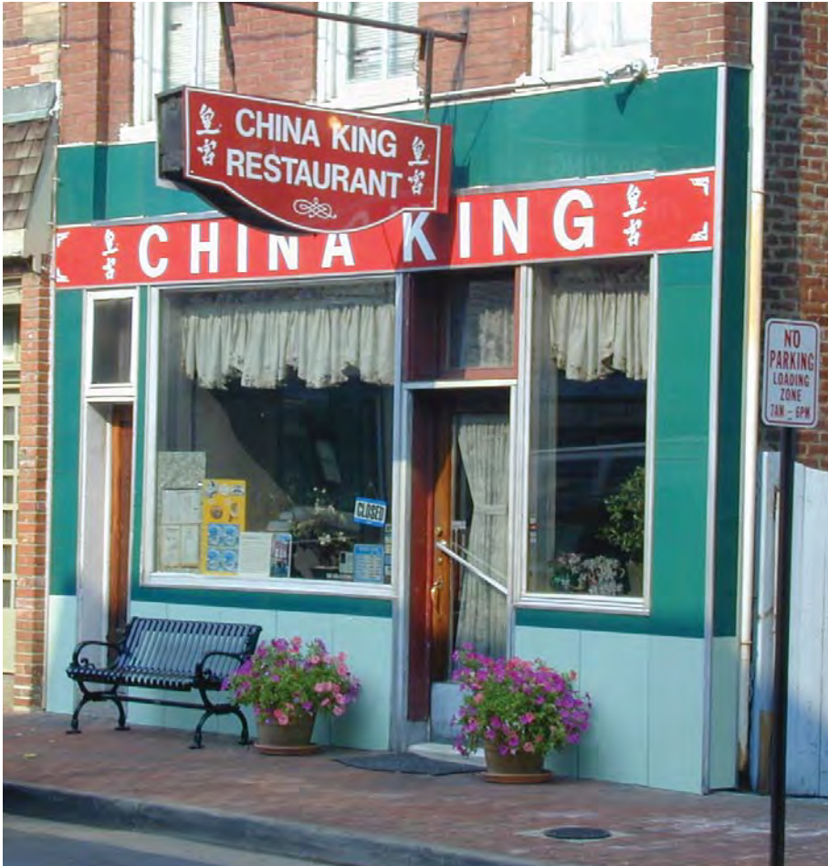
A recently rehabilitated example of a pigmented glass storefront. These glass panels in different colors were a very popular cladding for storefronts in the mid-twentieth century.
