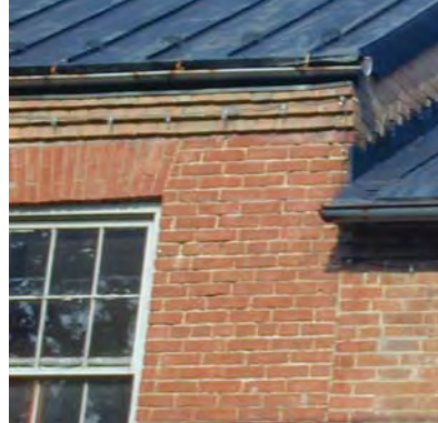
Two very different cornices on residential buildings: a classical dentilated cornice with modillions (left) and a simple, brick, corbeled cornice (above). Both are appropriate to the building's style.
