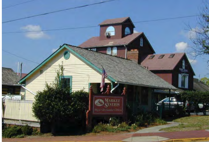
The Market Station complex is a successful reuse of a mill and accompanying outbuildings from Leesburg's past.
