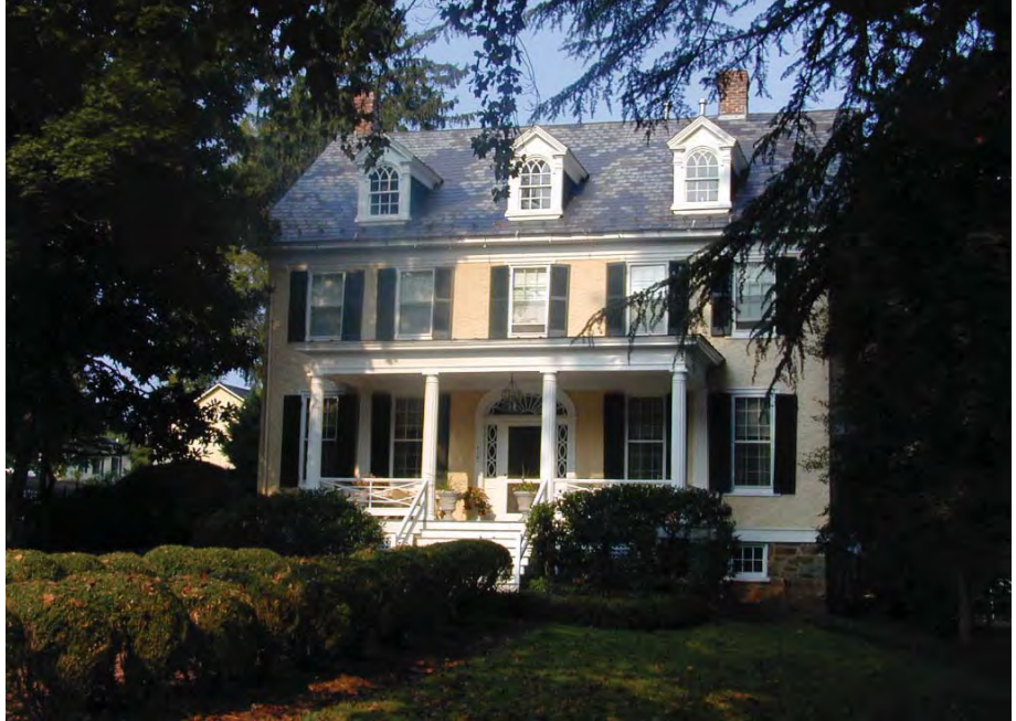
Large scale dwellings, such as this Colonial Revival example, are often located on larger parcels which allow for a deeper setback than seen on smaller lots in the neighborhood.
