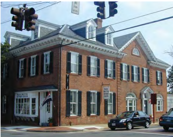
A hipped roof with a central gable and gable-roofed dormers.
