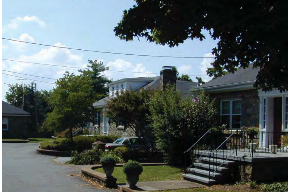
These Colonial Revival style cottages respect the traditional materials and details found elsewhere in the West Market Street Neighborhoods.
