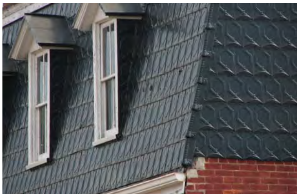
Stamped metal shingles were popular from the 1870s through the 1920s and are still manufactured today.
