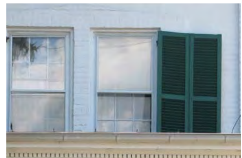
Paired windows may be shuttered by the use of a double-hinged shutter mounted to the outside of each window frame where it will not obscure the window opening.
