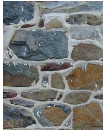
Stone, of various size and character, and with varying joint profiles, is used throughout the district for walls, foundations, and chimneys.
