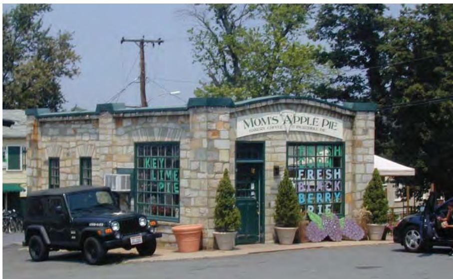
The vernacular style of the Esso Gas Station at the corner of East Market and Loudoun streets reflects the early architectural heritage of Leesburg through its use of stone jack arches with keystones over each opening.
