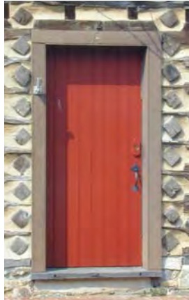
A vertical board door is appropriate for early vernacular styles such as this log structure.
