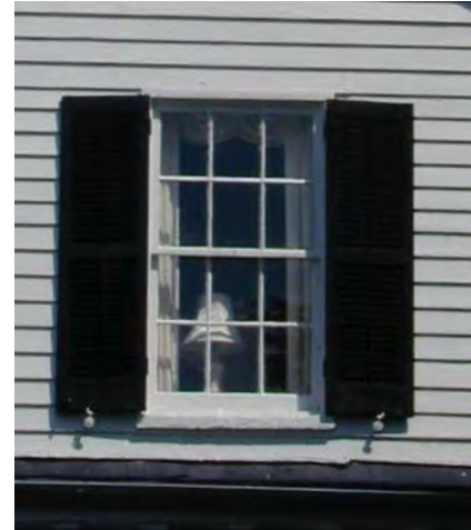
A window with shutters on a house with wood siding.
