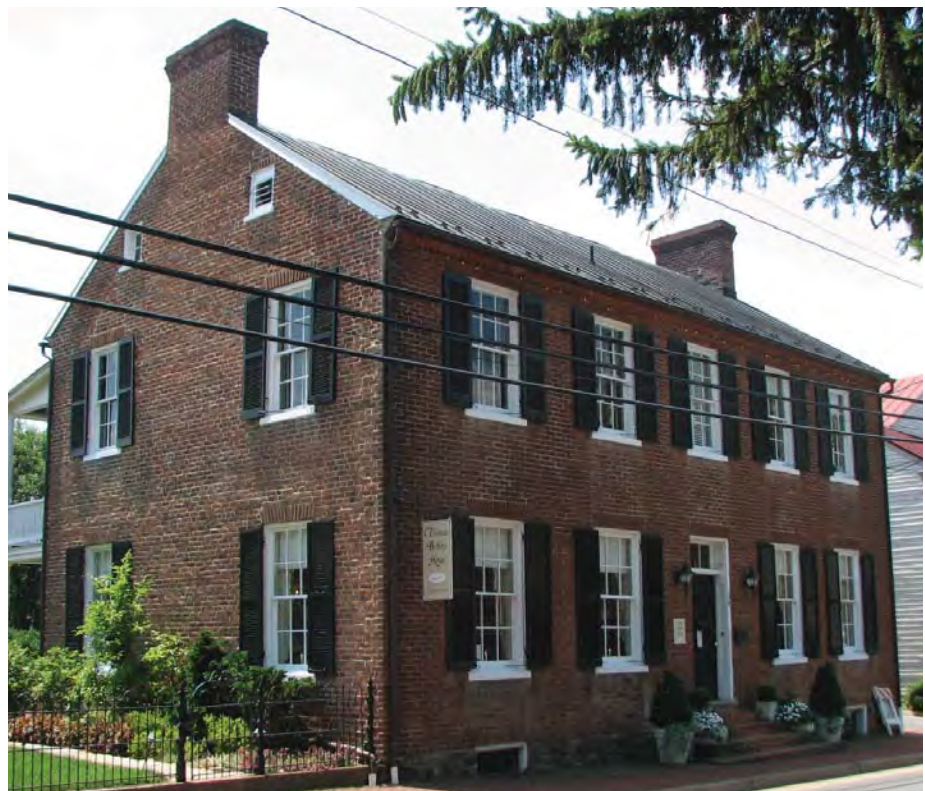
Located at 109 Loudoun Street, SW, this five-bay brick Georgian residence displays a symmetrical arrangement of openings, six-over-six light windows and a rectangular transom over the front door.
