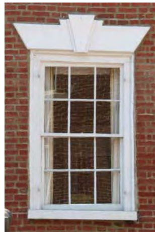
Six-over-six double-hung window.
