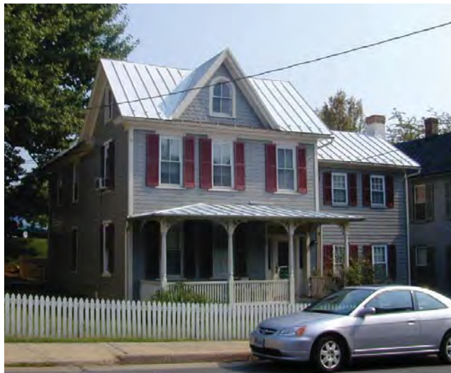
Additions to this Vernacular Victorian house include a rear wing and a side wing, both with appropriate massing, materials, and roof form.
