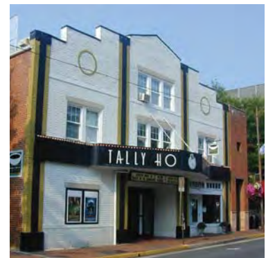
A canopy on West Market Street.
