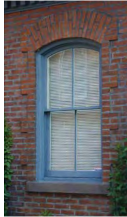
Two-over-two double-hung windows in masonry (above left and middle) and in wood siding with a decorative cap (above right).
