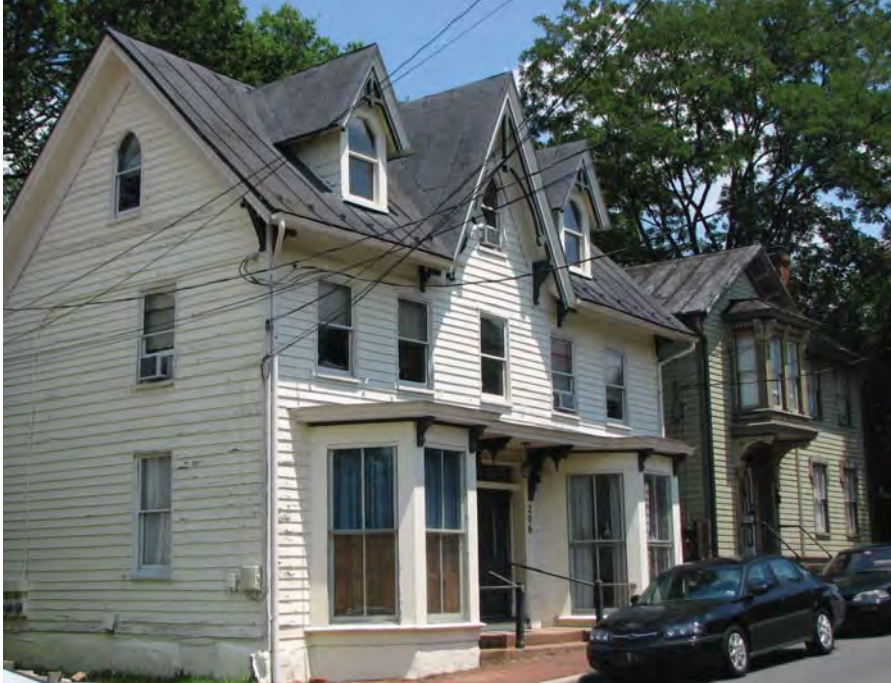
The steep central gable of this frame Gothic Revival residence is flanked by dormers that repeat the gable pitch and its decorative woodwork. Note the Gothic arched attic window in the gable end.
