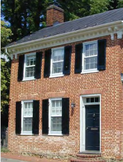
This Federal-style brick dwelling represents early settlement in a West Market Street neighborhood. The brackets at the cornice indicate a Victorian update of the facade.
