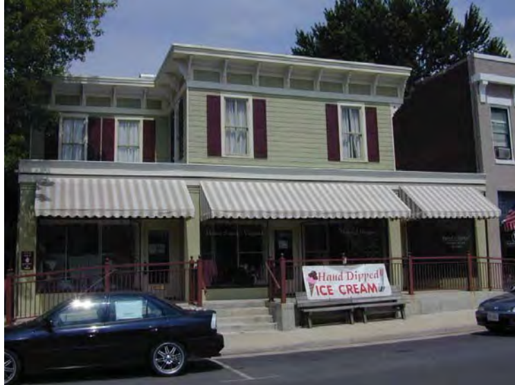
This new accessible entrance to a traditional commercial building uses the topography of the site to help make up the difference in grade.
