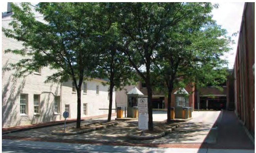
The entrance to Leesburg's municipal garage is landscaped to soften the appearance of the structure.
