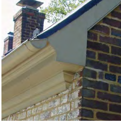
A simple wood cornice and boxed eave.
