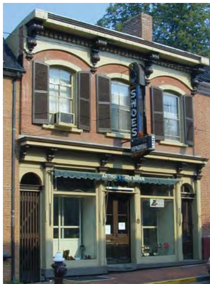
The building cornice and storefront cornice on this downtown building use the same brackets and colors to unify the design.
