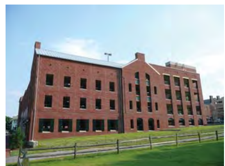
The design of the Sophia Street parking garage in Fredericksburg uses a variety of techniques to reduce its overall mass such as a different design for each of its three bays.
