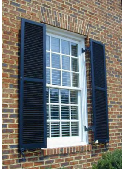
Operable shutters with typical hardware are shown here on a masonry wall.
