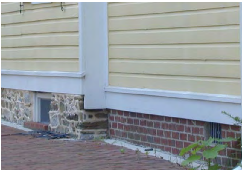
(below) A building with a stone foundation and an addition with a brick foundation, the two most common foundation materials in Leesburg.
