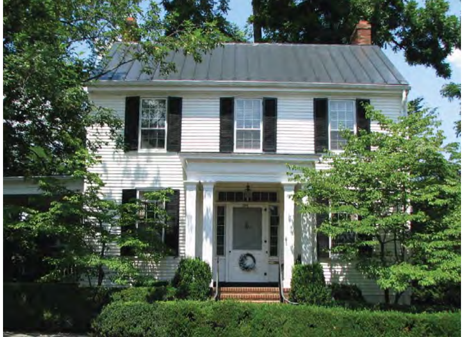
The facade of this frame Greek Revival style house is accentuated with a classically-designed portico, and multi-paned sidelights and a rectangular transom framing the front door.
