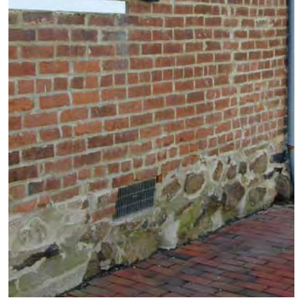
A stone foundation on a brick building.
