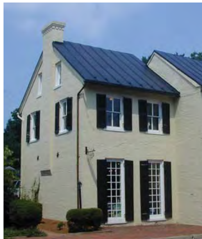
A metal side gable roof.
