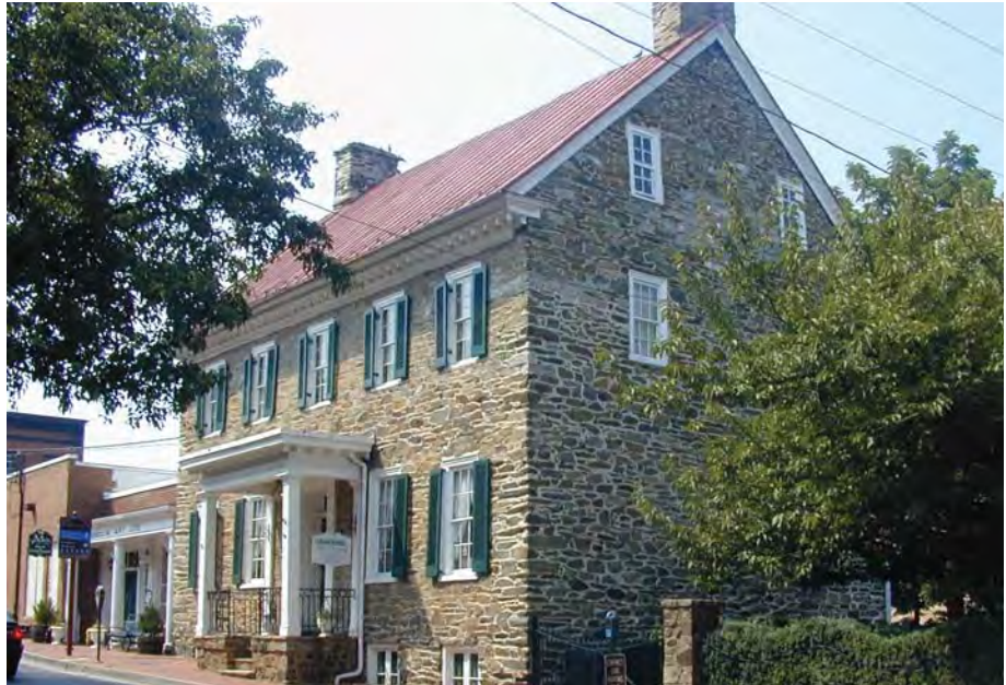
A heavy modillion cornice accentuates the facade of this five-bay Georgian fieldstone dwelling.
