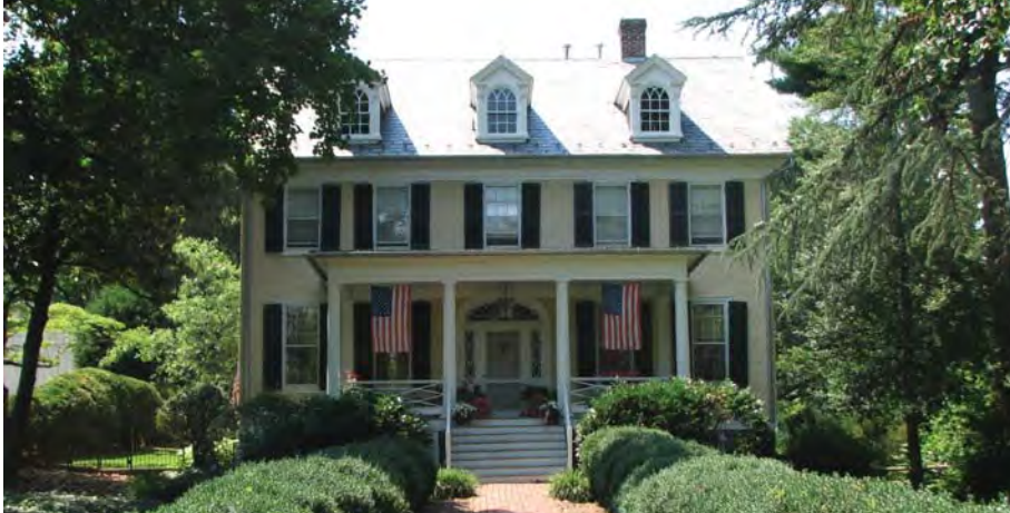
This symmetrical stone Colonial Revival dwelling repeats classical details, such as the door surround and fanlight and small-paned windows, characteristic of the Georgian and Federal architectural styles.
