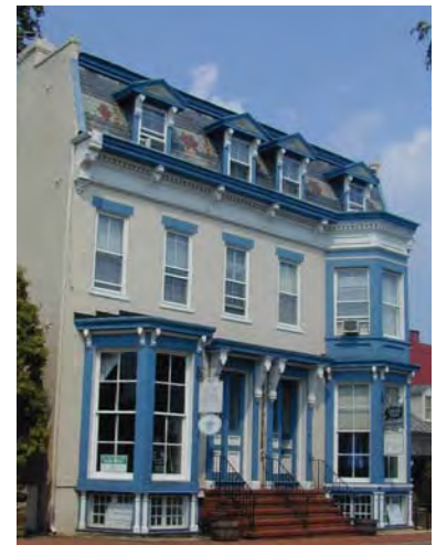
A mansard roof.
