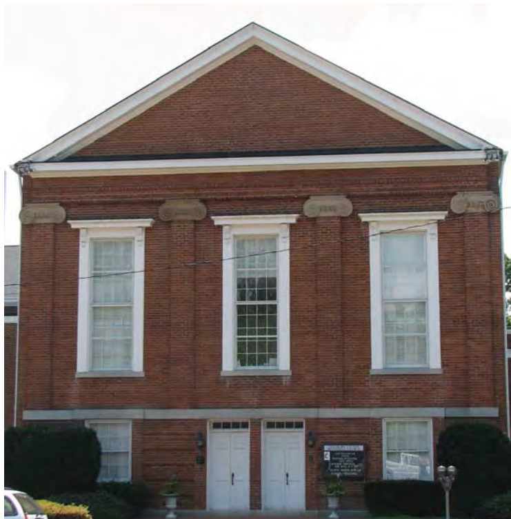
The temple-front Presbyterian Church on West Market shows a religious adaptation of the Greek Revival style with Ionic pilasters adorning the bay divisions between the twenty-over-twenty light windows capped by bracketed window hoods.
