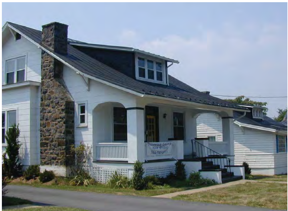
The long sweep of the gable roof on this bungalow contains the porch as well as a shed-roofed dormer. Note the deep overhang of the eave and the simple brackets that appear to support the roof.
