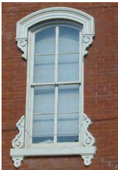
An arched four-over-four double-hung window with decorative scrollwork.
