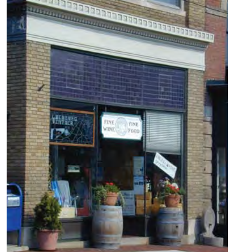
A metal storefront with prismatic glass transom.
