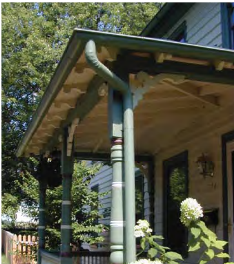
A wood porch with turned columns, decorative brackets and exposed rafter tails.
