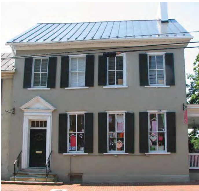
This three-bay Federal-style dwelling features Flemish bond brickwork and jack arches over the window and door openings.
