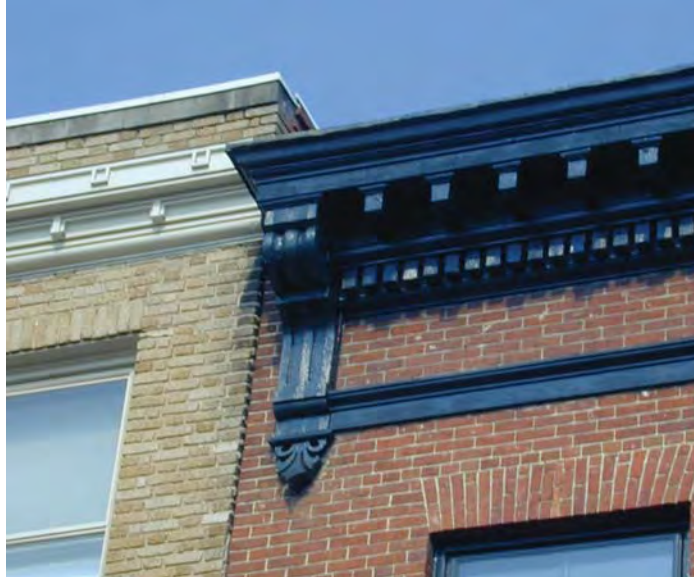
An Italianate commercial cornice, featuring wood brackets, dentils, and modillions.
