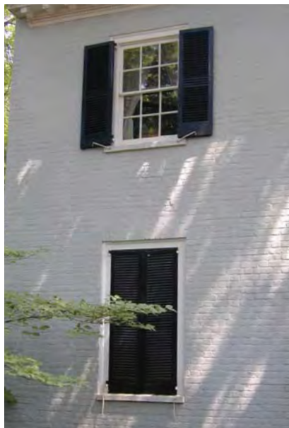
Operable shutters allow the control of light and air.
