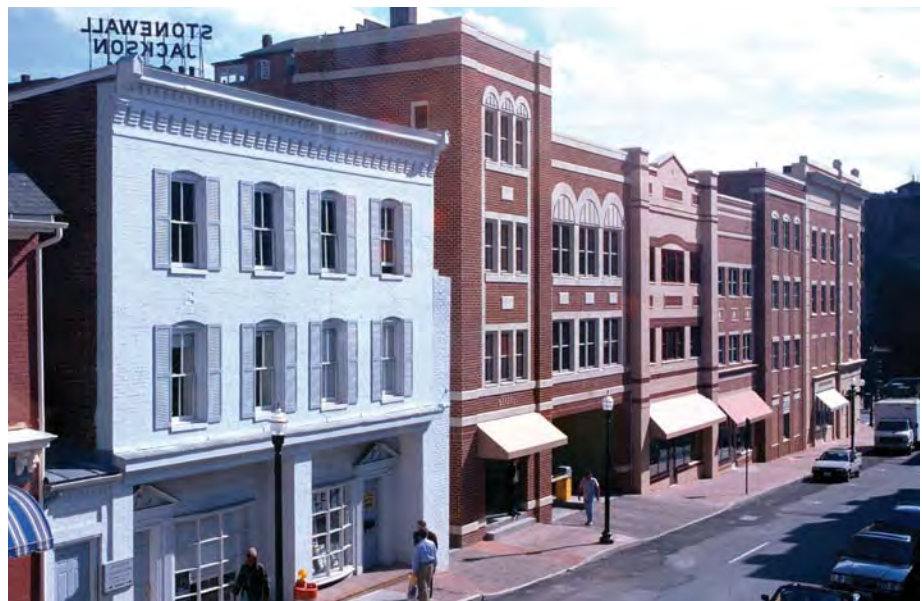
Storefronts, highlighted by awnings, were incorporated into the design of the parking garage in Staunton, VA to relate the new construction to the historic context of the streetscape.
