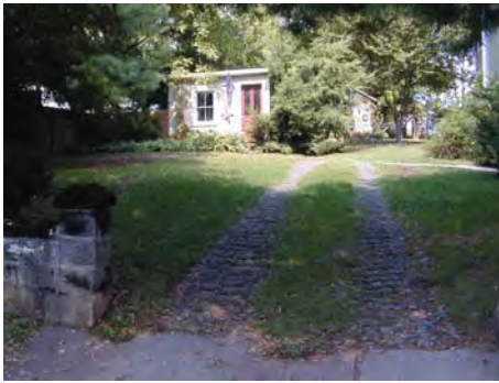
Ribbon concrete and stone driveways are common in the district and should be retained.
