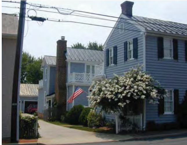
The large addition to this residence is placed behind the original building and does not impact the orientation of the original house.
