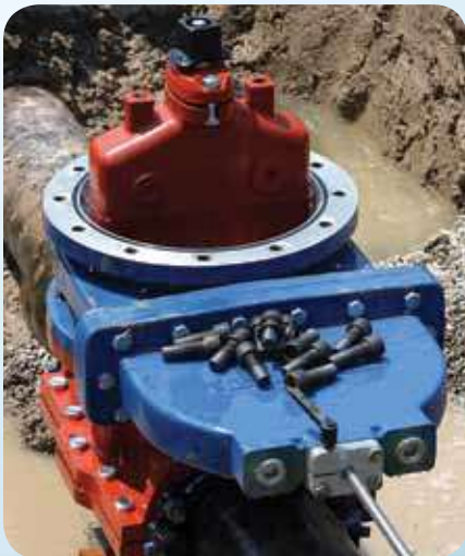
Low-profile bonnet used as line stop.
