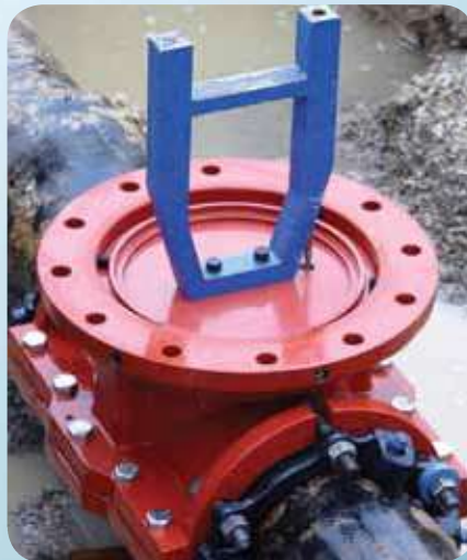
Internal equalization completion plug installed.
