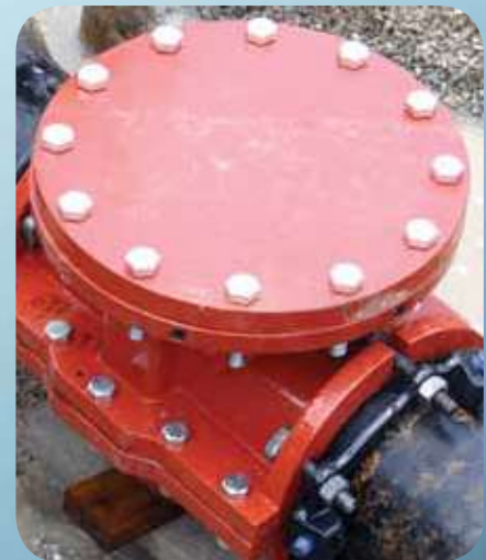
Blind flange installed.
