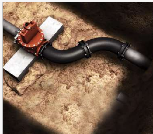
Step 6 Connect new pipe.
