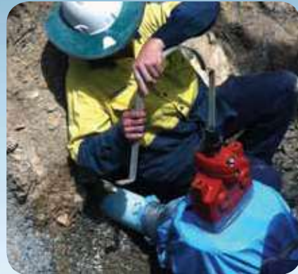
An InsertValve installation under full line pressure.
