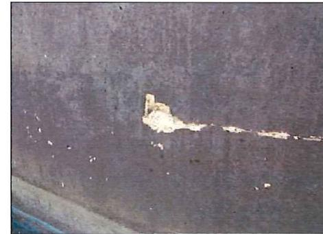
INTERIOR CONCRETE WALL COATING DELAMINATION
