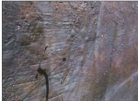
INTERIOR CONCRETE WALL COATING BLISTERING
