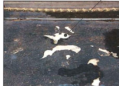
COATING FAILURES AT CONCRETE FLOOR
