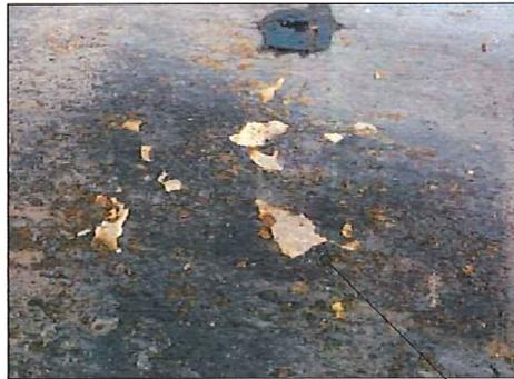
COATING FAILURES AT CONCRETE FLOOR
