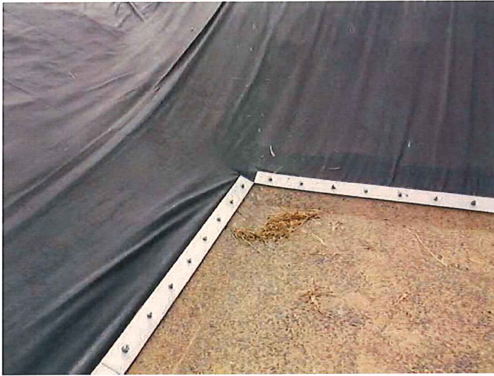
10) Aluminum strip securing bottom of liner.
