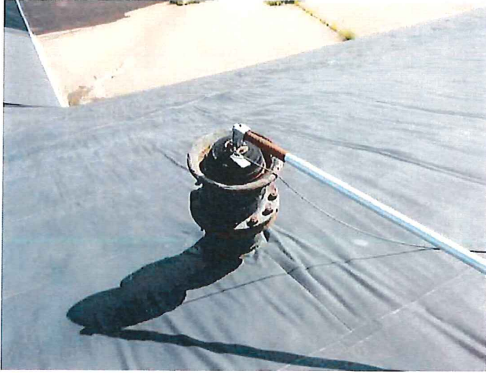
4) Pipe penetrations in wall liner.
