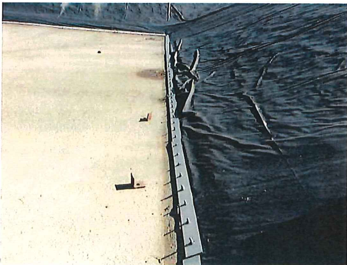
6) Liner secured with aluminum strips and bolts at concrete floor.
