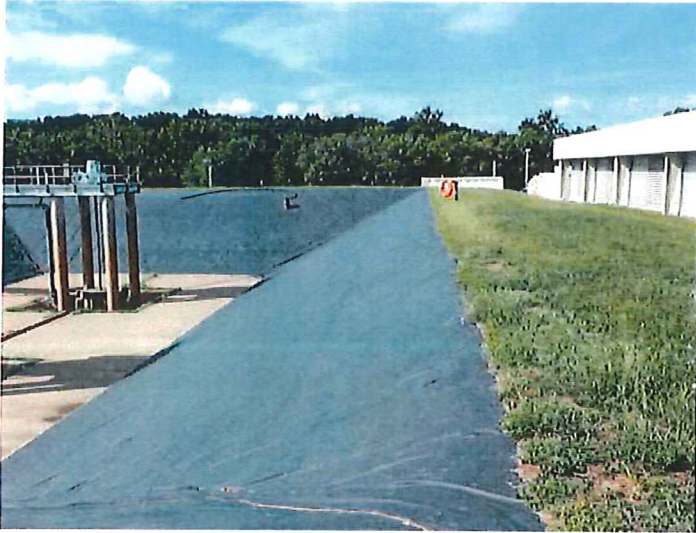
1) Rubber liner on dirt sloped walls.
