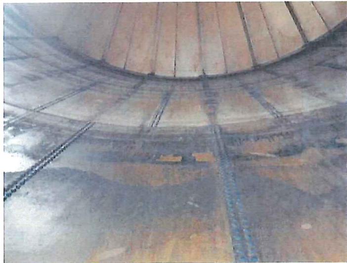
35) Sidewall coating is in fair condition.
