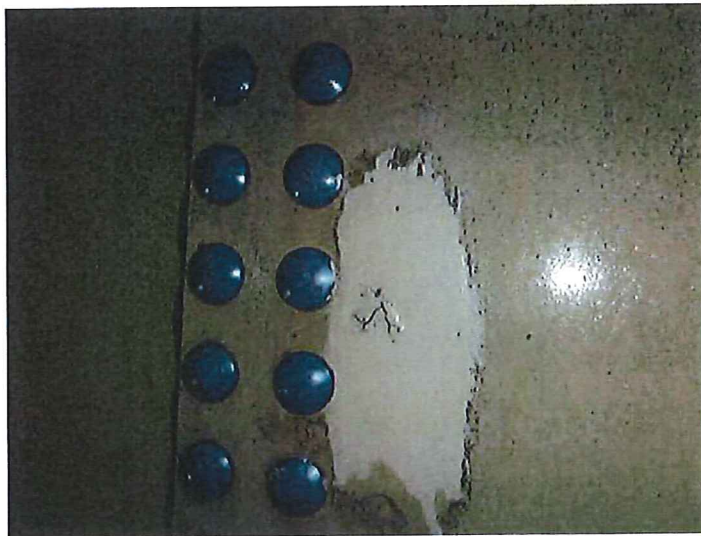
33) Coating repair made on the sidewall.
