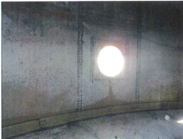
27) Sidewall manway viewed from interior.
