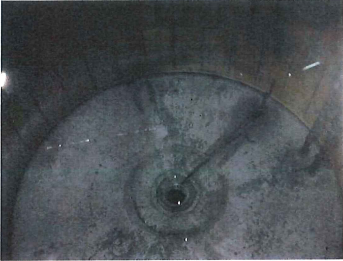
25) Concrete floor is in good condition.
