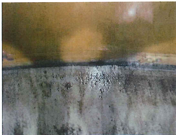
36) Floor to sidewall connection is in good condition.
