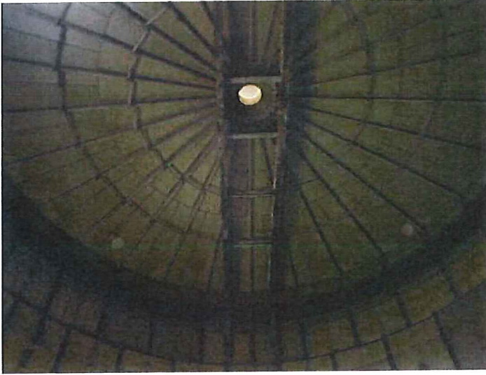
28) Bolted steel roof with radial stiffeners.
