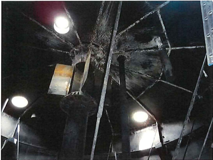
28) Interior cap with support structure.
