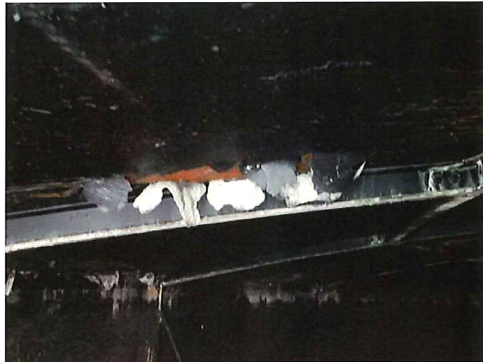
32) Interior roof cap with coating failures.
