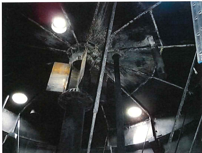
15) Roof cap with stiffeners.
