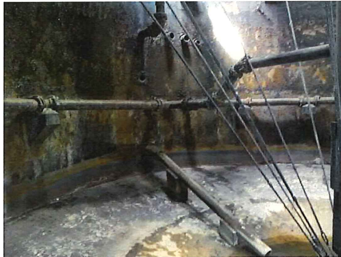
17) Interior piping coating is in fair condition.
