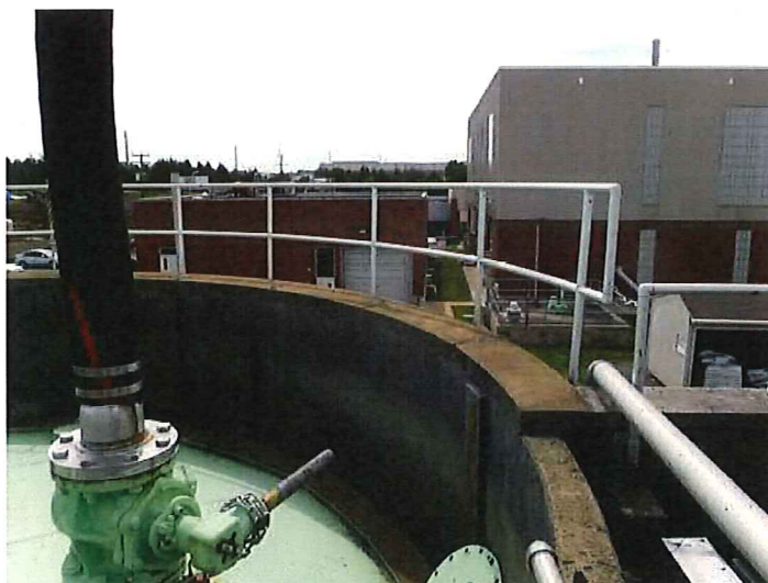
12) Roof cap is on a roller assembly attached to interior of sidewall.
