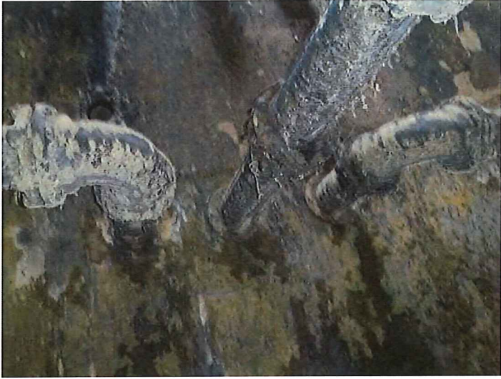
19) Sidewall coating around piping.
