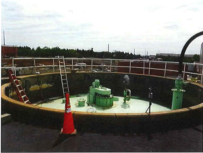
7) Outside of floating roof cap.
