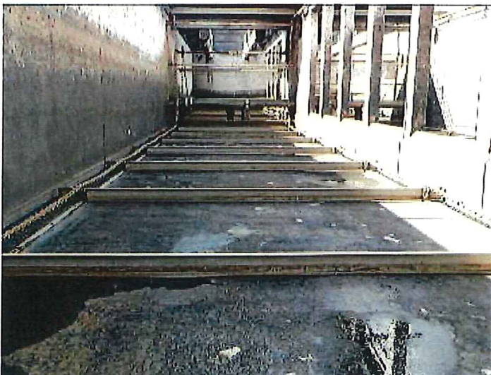
18) The sludge scrapers are in good condition.
