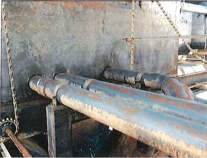
16) The piping is in good condition.
