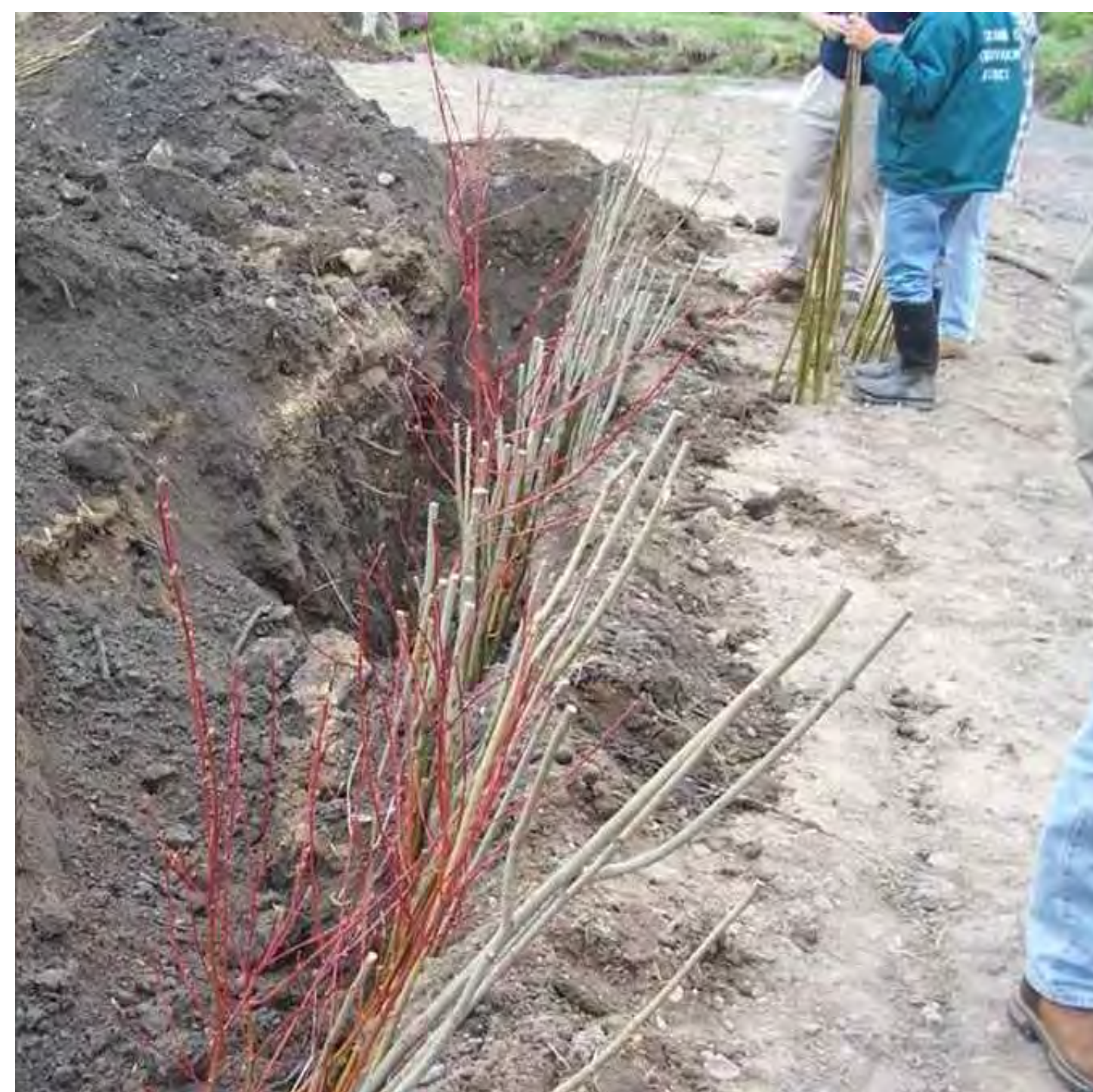
EXAMPLE SLIT TRENCH (SHOWN FOR INFORMATION ONLY)
