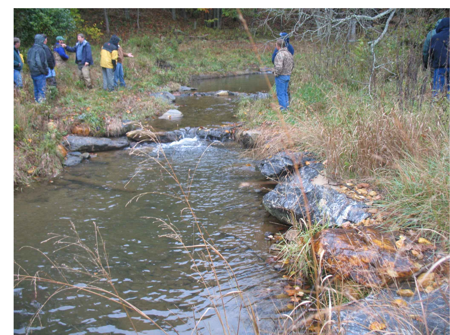
EXAMPLE CROSS VANE (SHOWN FOR INFORMATION ONLY)
