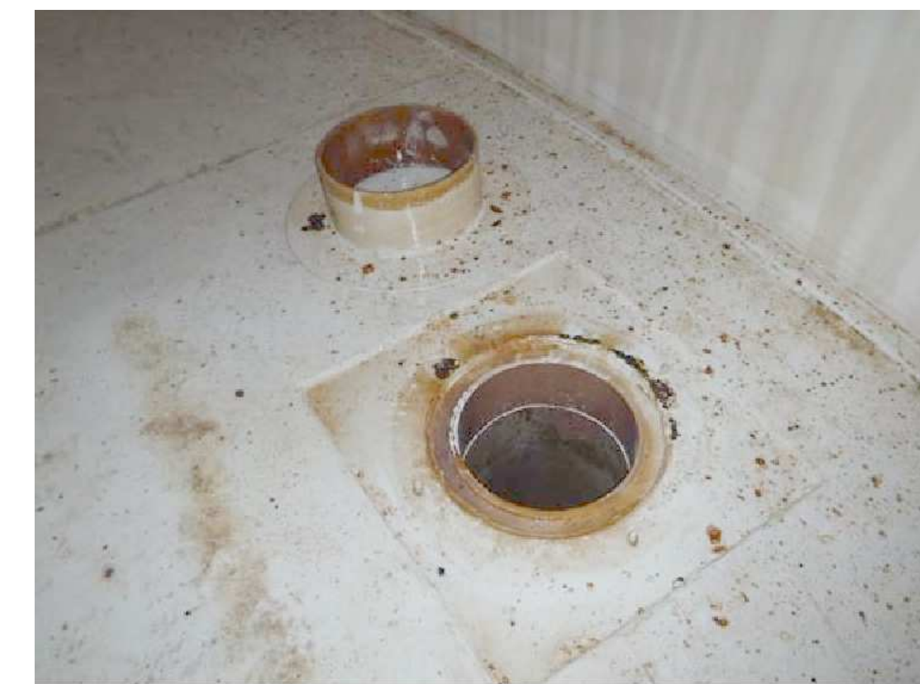
FILL PIPE STUBS AT FLOOR NO SCALE
