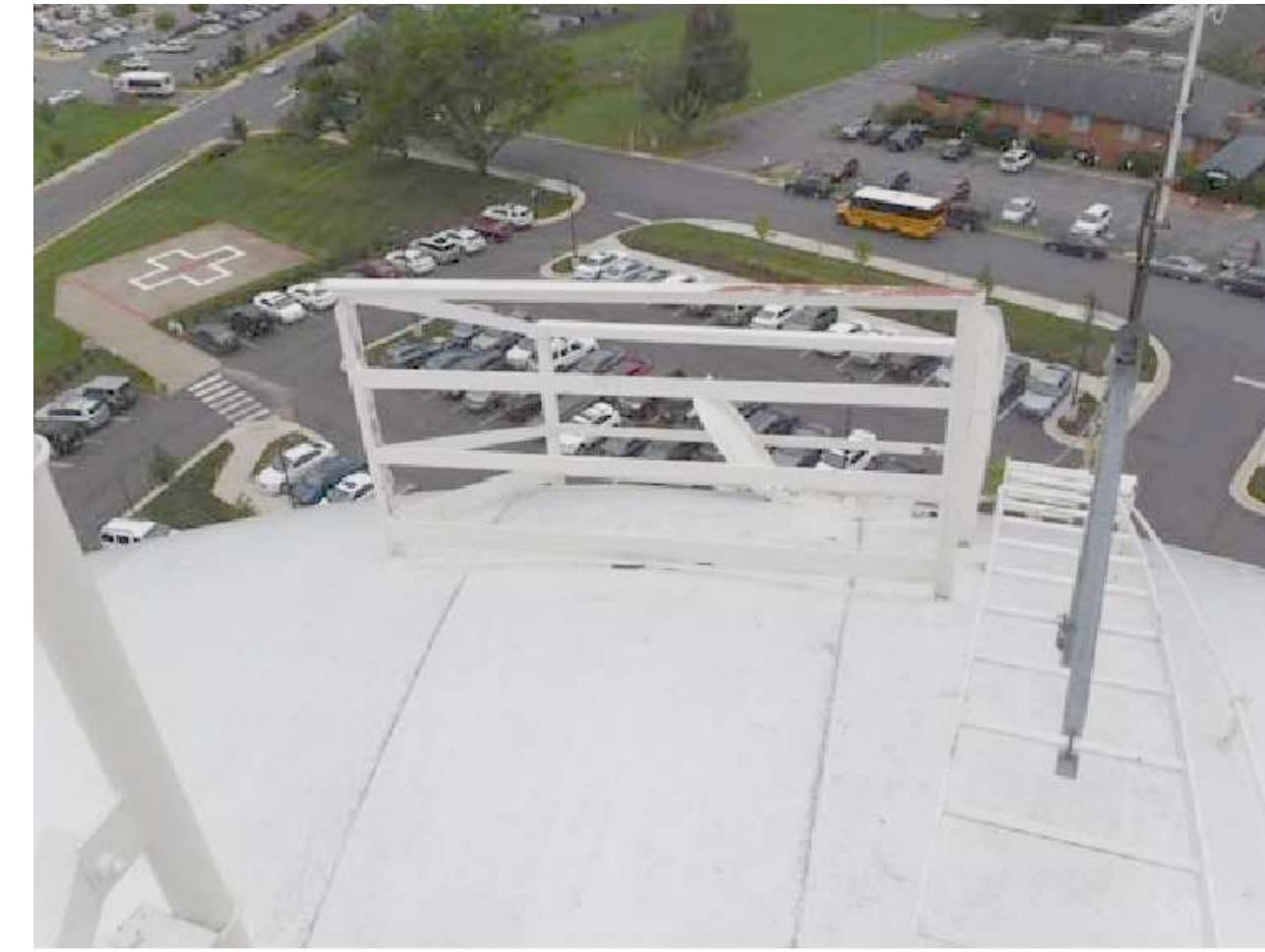
HANDRAIL AROUND ROOF HATCH NO SCALE
