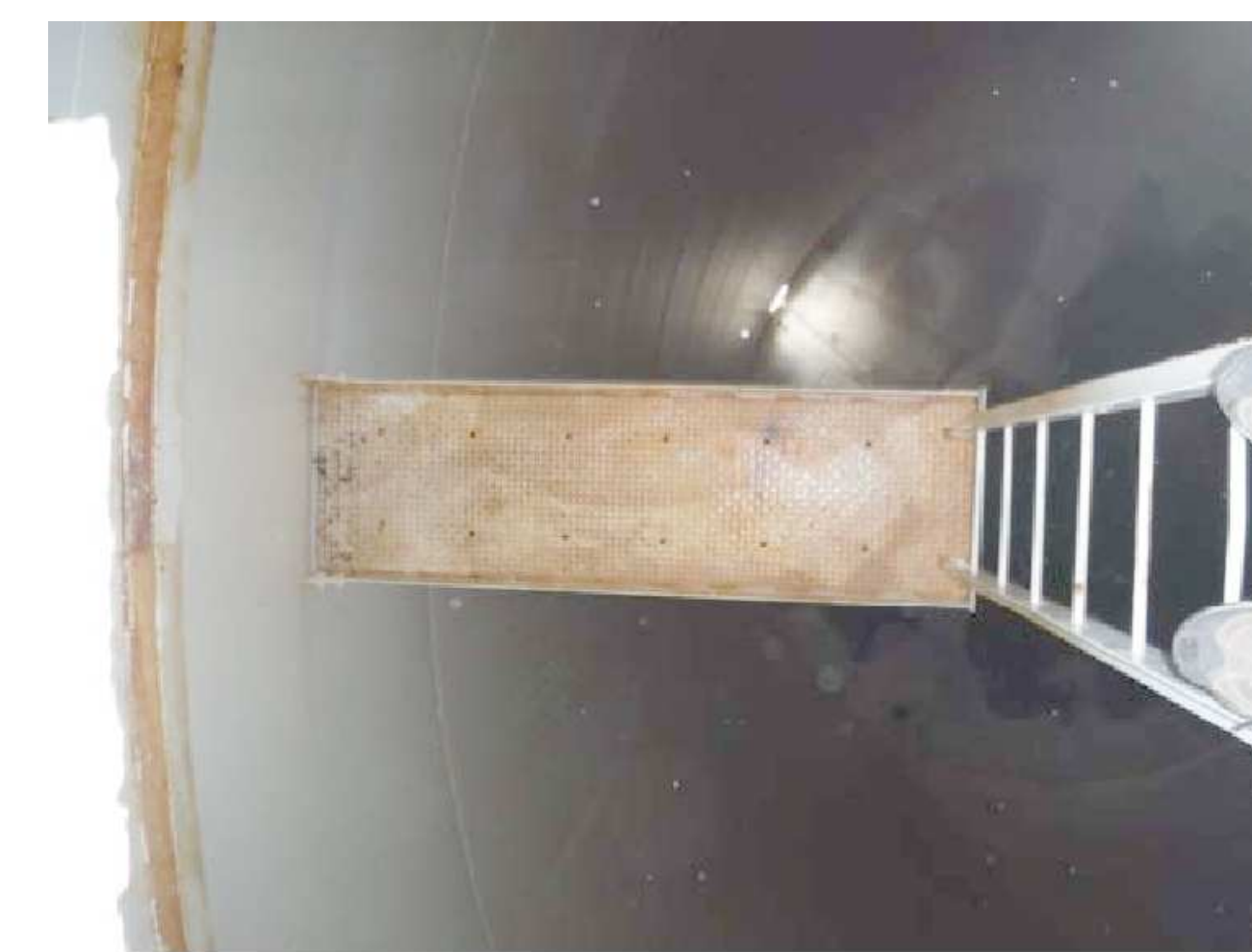
PLATFORM APPROX. 12' BELOW ROOF HATCH NO SCALE
