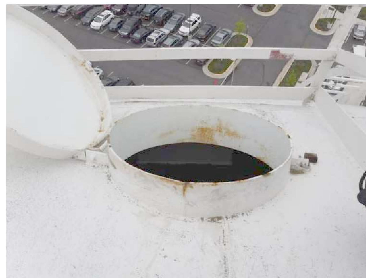
ROOF HATCH NO SCALE
