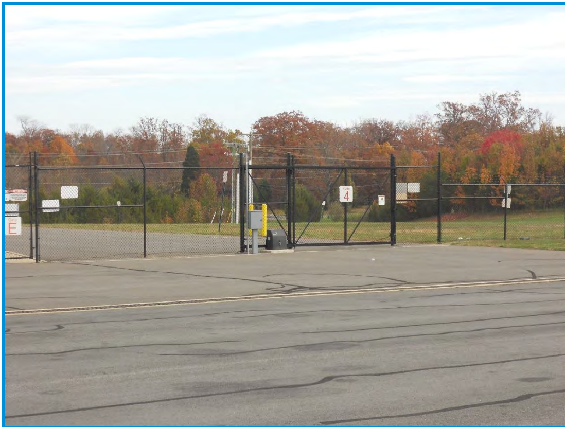
Exhibit 1-15 JYO Access Gate
