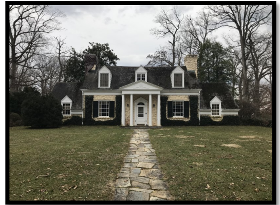
Historic 1937 manor house at White Oak
