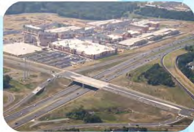
New Route 7 interchange at River Creek Parkway & Crosstrail Boulevard
