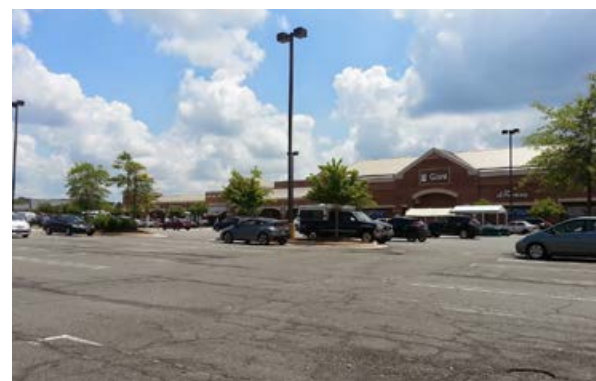
Some older retail centers lack the character that contributes to the desired Leesburg brand.
