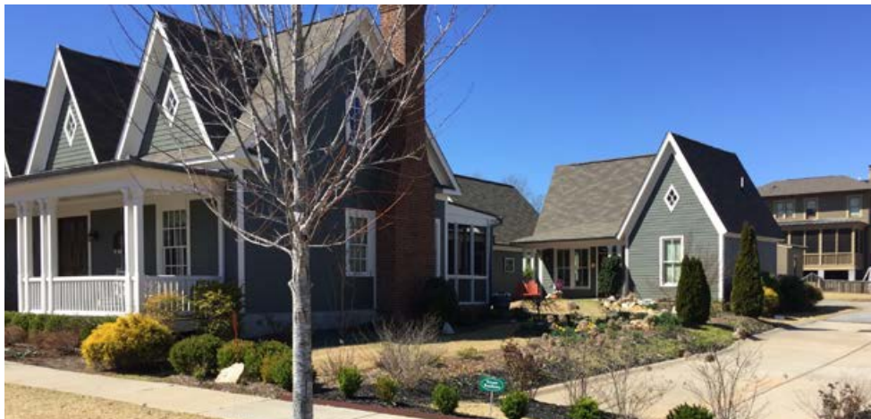
Accessory Dwelling Units help support housing costs and provide a greater range of housing options.
