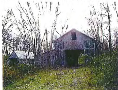
Figure 23: Existing corn crib in Zone 5, the riverfront support zone.
