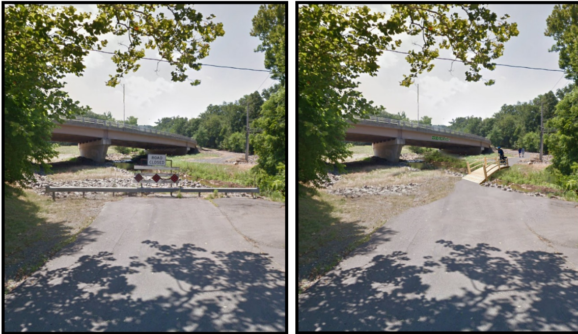
Figure 4. Existing W&OD Trail / Sycolin Road Overpass (left) and Rendering of Multiuse Path
