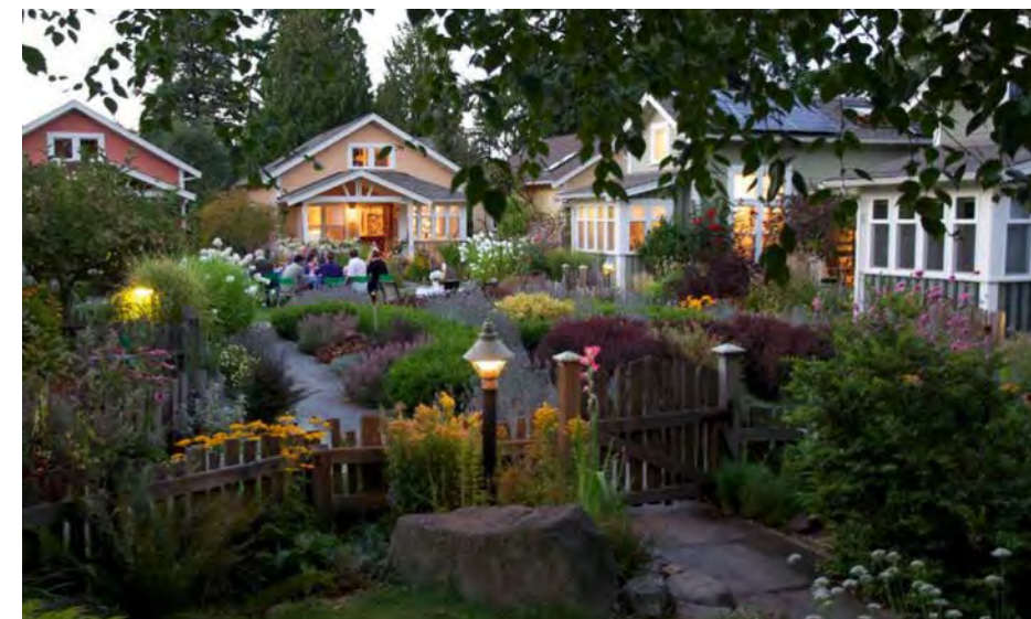
“Cottage court” development in a suburban setting to address economic diversity and enable older residents to age in their community.
