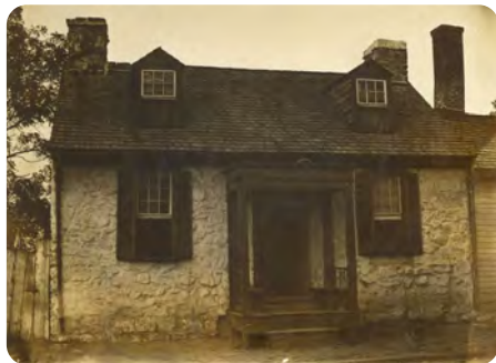
William Baker's House One of the original buildings in Leesburg
