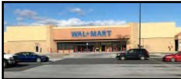
Above: Building prior to renovation
