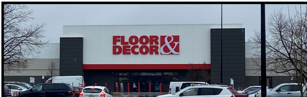
Below: Building after renovation
