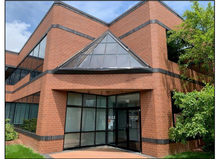
Remote Tower Center Building
