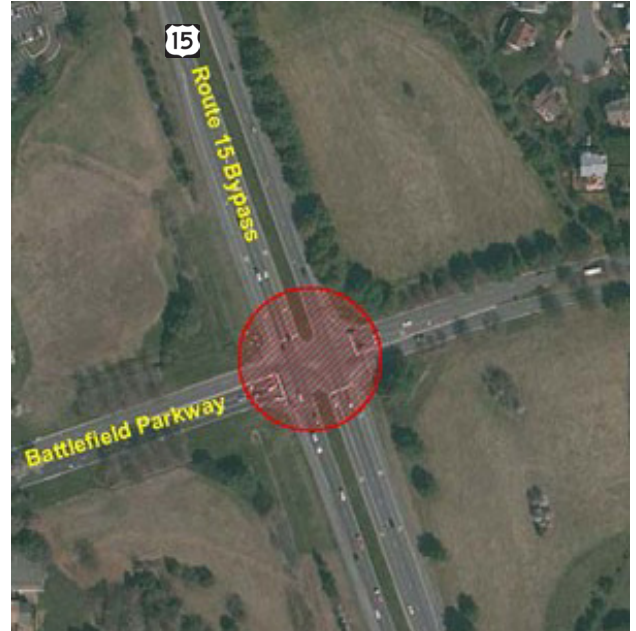
Route 15 Bypass and Battlefield Parkway - Town of Leesburg, VA
