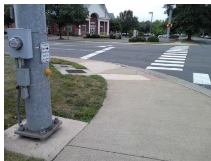
Catoctin Circle & Harrison Street: No locator tone, vibro-tactile indication, or speak walk message at the signal. The push button distance is not compliant.
