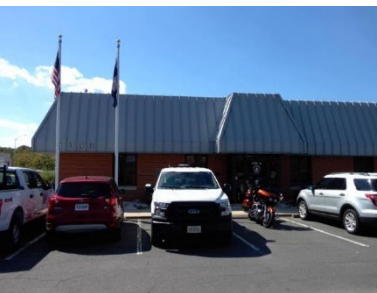
Town Maintenance Building
