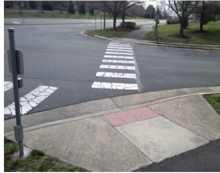
Kincaid Blvd SE & Patrice Drive SE: The width of the crosswalk is not compliant.
