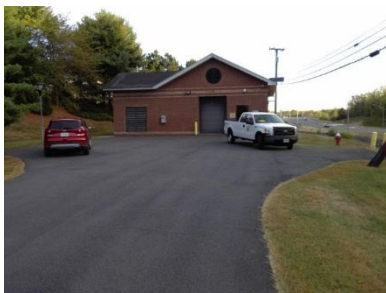
Utility Pump Station
