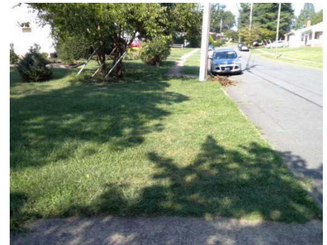
Prospect Drive SW: A section of sidewalk is missing and consists of dirt, grass or gravel.
