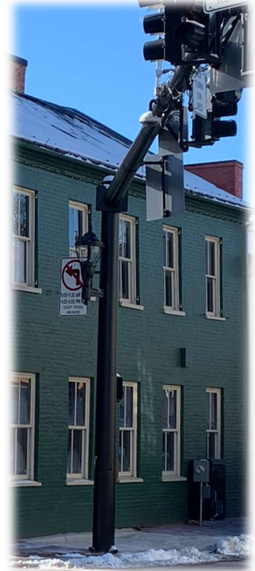
Mast Arm Light
