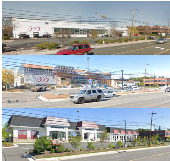
Recent facade improvements and changes in land use transformed the old Loudoun Motor Sports Dealership into a jewelry store, salon and restaurant and demonstrate how incremental changes can help transform commercial corridors into more walkable areas that serve nearby residents and draw character from the Old and Historic District.
