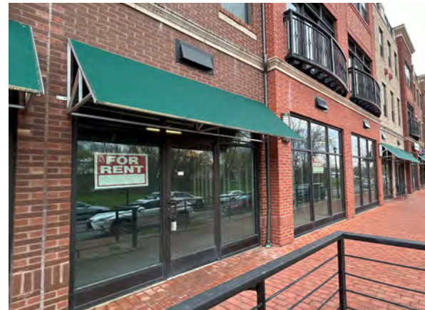
Storefronts in the Crescent Place development are currently vacant as the retail market struggles.
