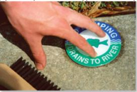
Finish Step on disc to use body weight to embed disc into adhesive. You have now successfully installed a storm drain marker!
