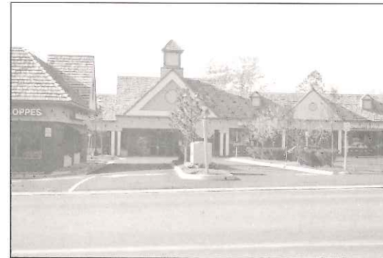
A planted median makes entry drives more attractive and promotes safer crossing for pedestrians.
