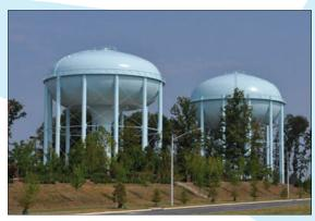
provide redundancy within the system, allowing tanks to be taken out of service for maintenance without affecting service to customers. Both new water tanks have been included in the Town's Utilities Master Plan since 1987, although not with specific locations.
